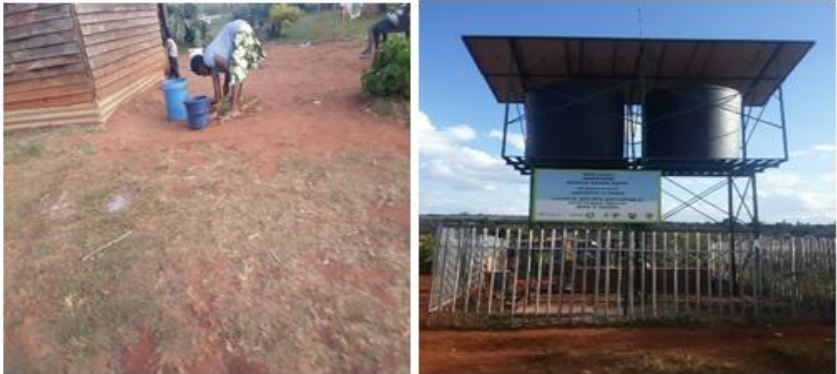
Plate 2: Water facilities in Magamba, Hatcliffe Extension (Field survey, 2022)
