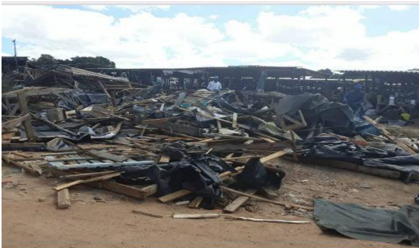
Figure 1: Market sheds being demolished by the City Council.
